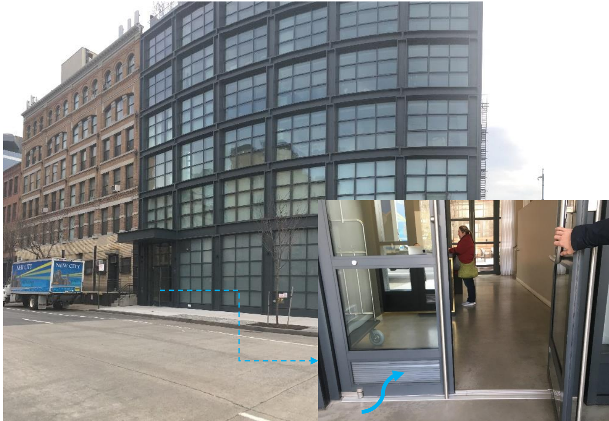
Residential Building with access at grade (wet-floodproofed)
